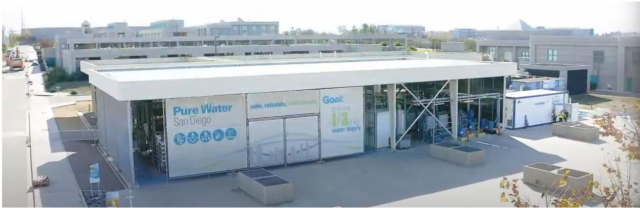
Figure 4-1: North City Demonstration Pure Water Facility
