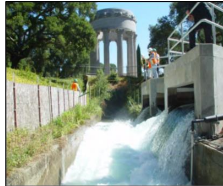
Above: Flows from the Pulgas Dechloramination Facility enter the Pulgas Discharge Channel for release to Upper CSR.
