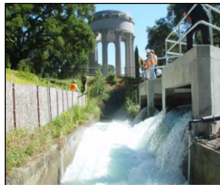
Above: Flows from the Pulgas Dechloramination Facility enter the Pulgas Discharge Channel for release to Upper CSR.
