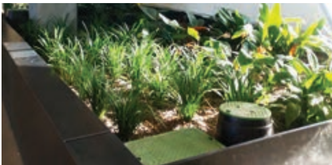
2nd stage of wetland treatment in building's interior (image courtesy of Denver Water)
