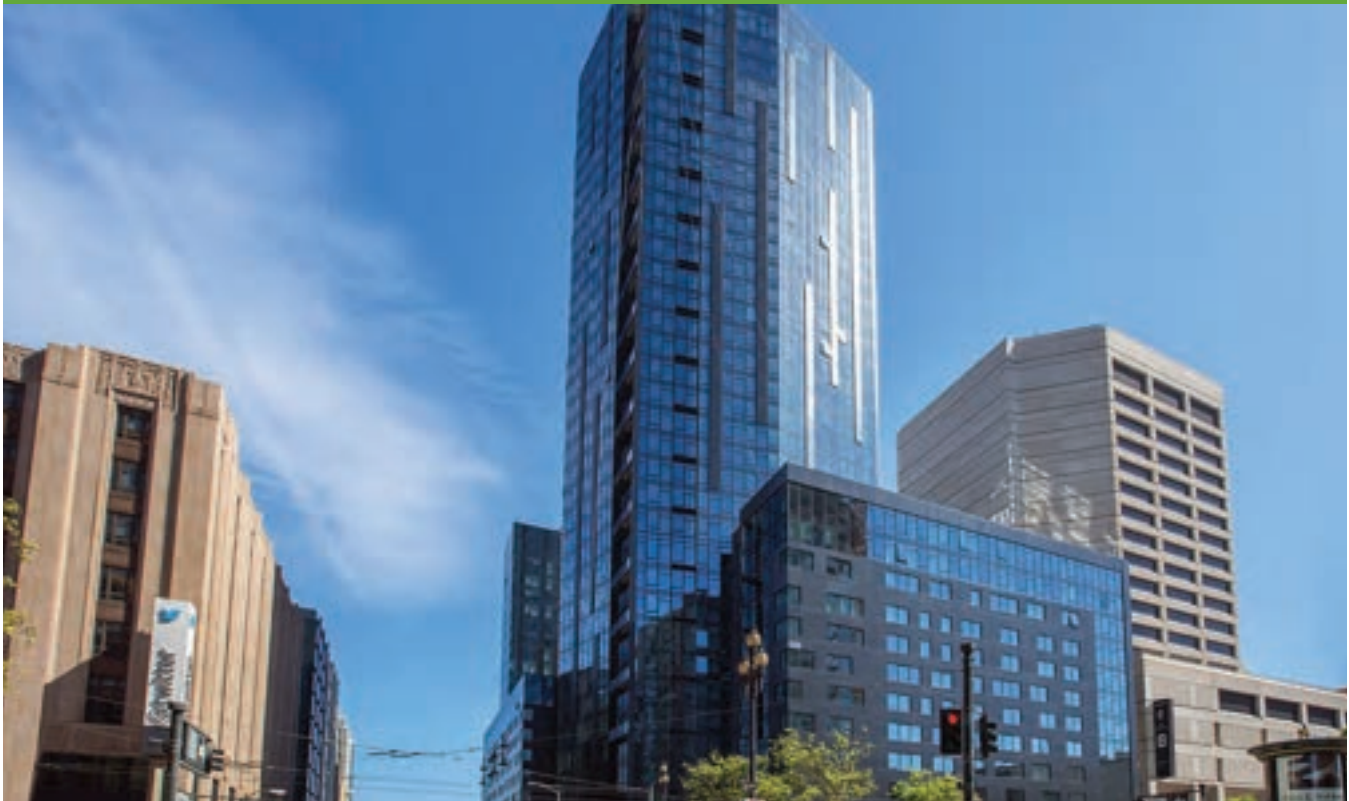
NEMA apartment complex (image courtesy of Epic Cleantec)
