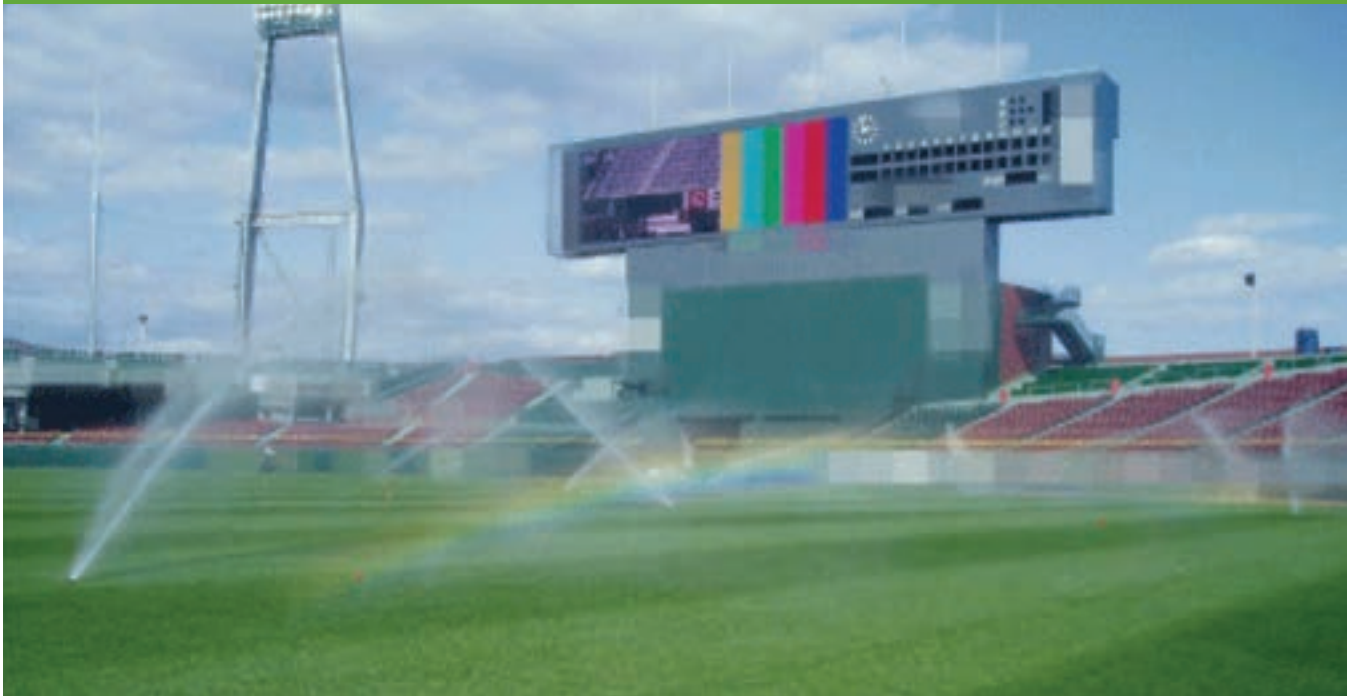
The baseball field's rainwater fed sprinkler irrigation system (photo source: www.city.hiroshima.lg.jp/site/gesuido/2638.html )
