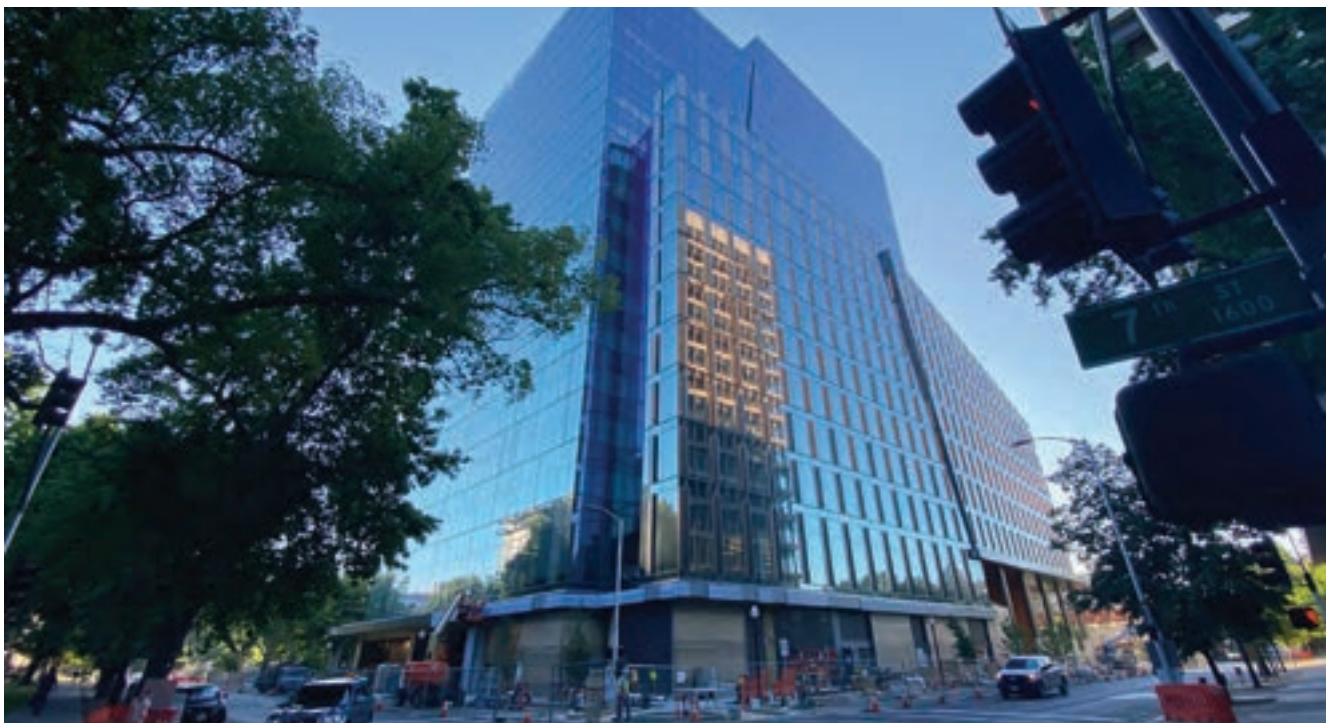
DGS Natural Resources Building in Sacramento, CA will capture graywater, treat, and reuse it for toilet flushing. (Image courtesy of HTEC)
