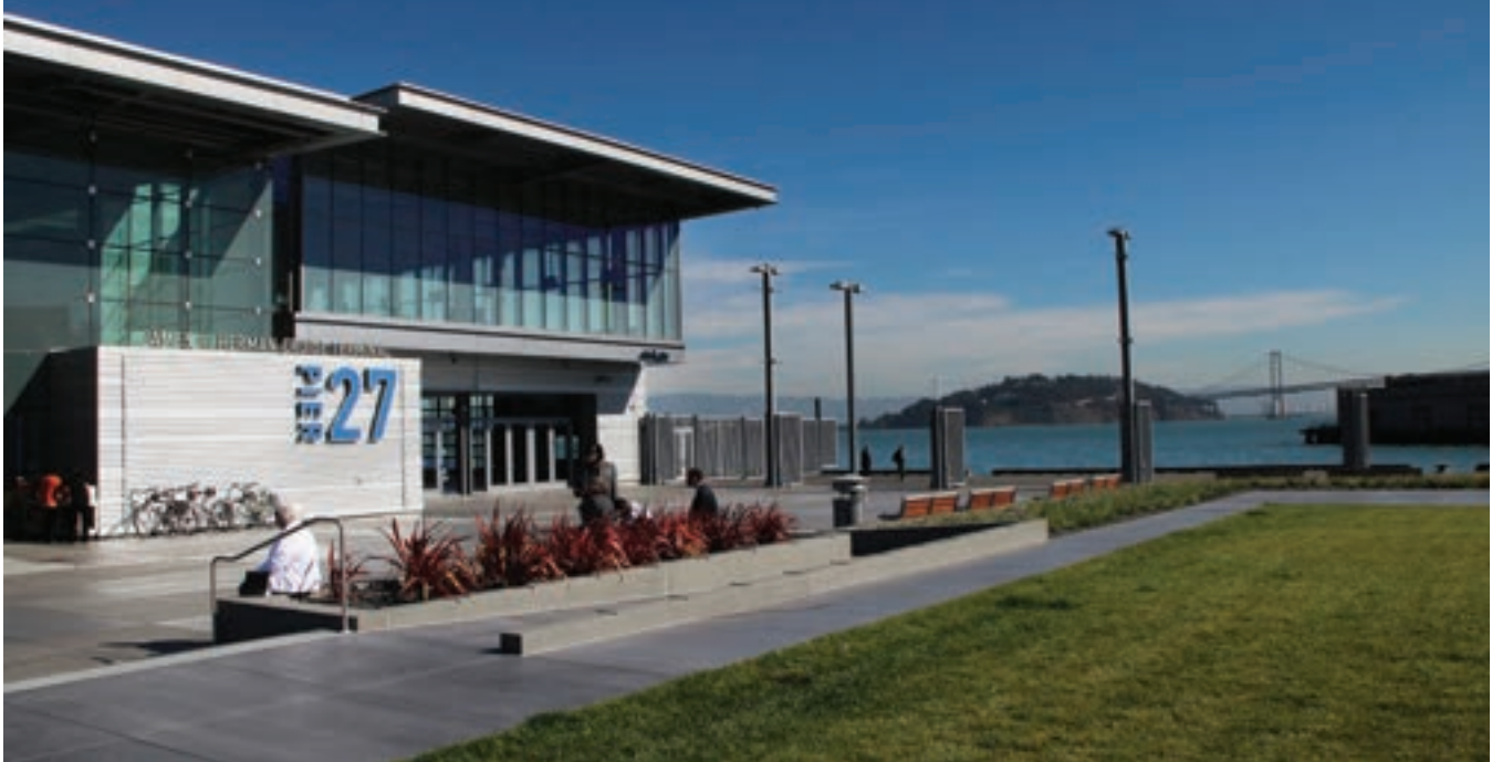
The James R. Herman Cruise Terminal at Pier 27 (image courtesy of San Francisco Public Works)
