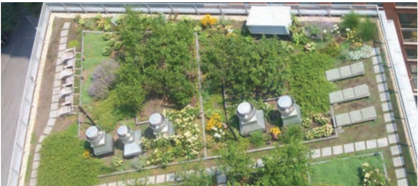
The green roof reduces runoff, insulates the building, and is irrigated by the onsite reuse system (image courtesy of NSU)
