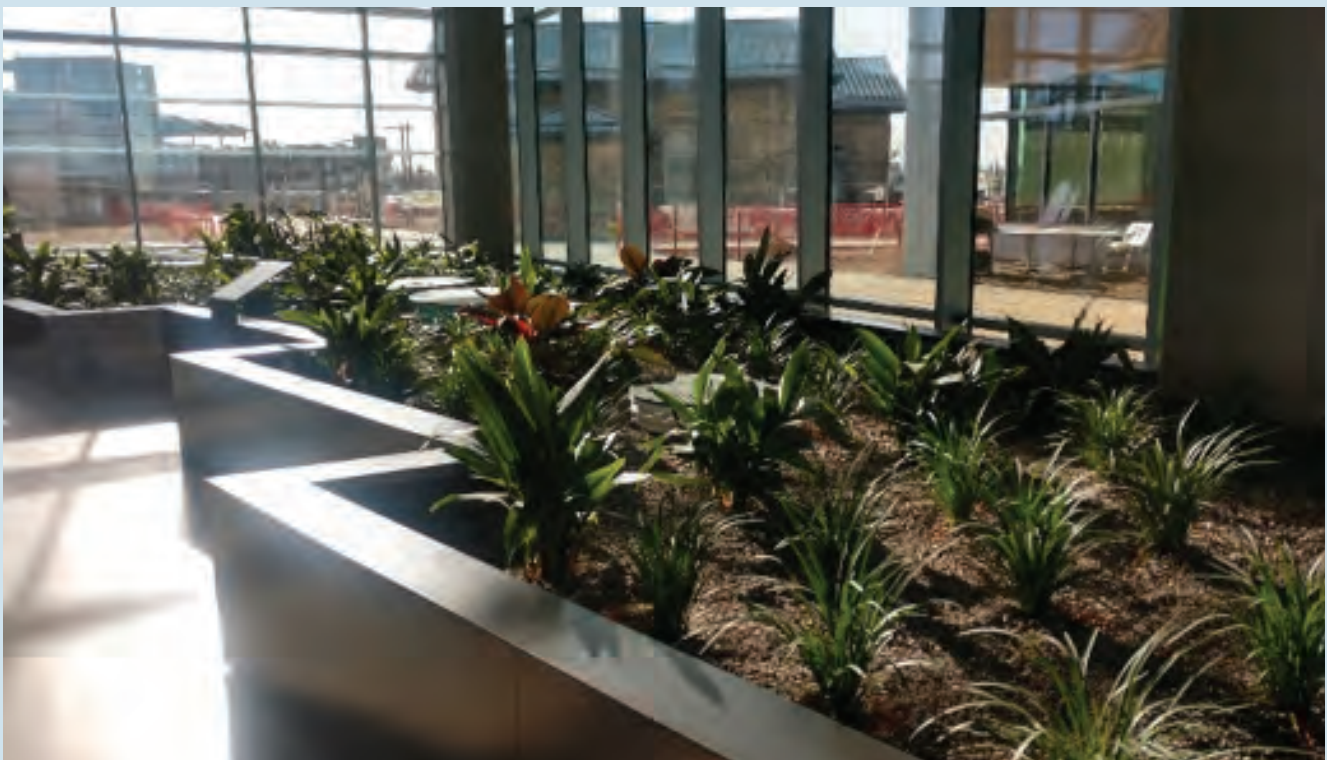
Denver Water's Wetland System Treating the Building's Blackwater in Denver, CO (image courtesy of Denver Water)
