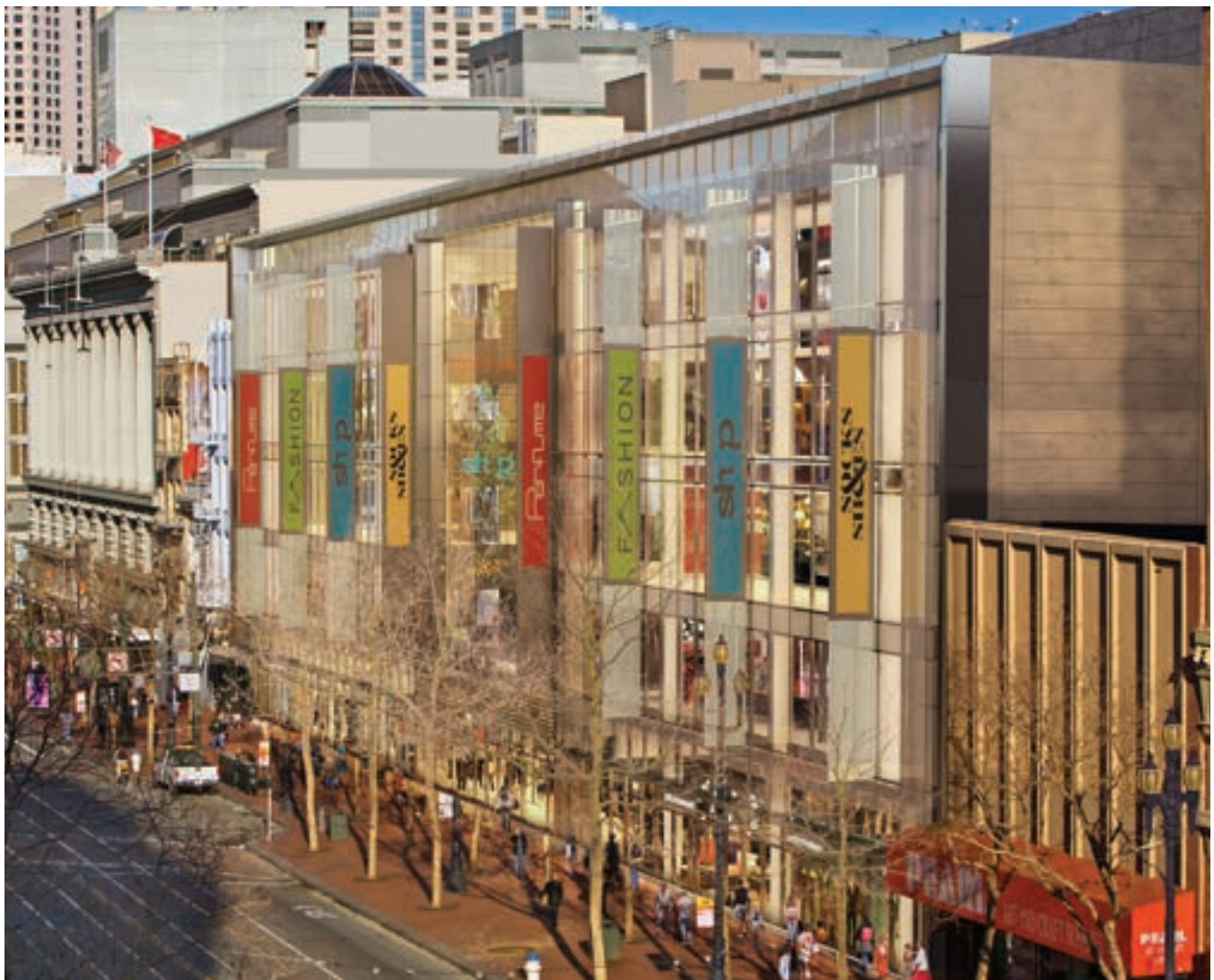
Market Street Place (image courtesy of CRP/Cypress Market Street, LLC)
