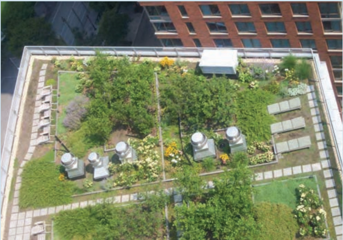
Green Roof of the Solaire Building Which Recycles Its Blackwater Onsite in New York City (image courtesy of Natural Systems Utilities)
