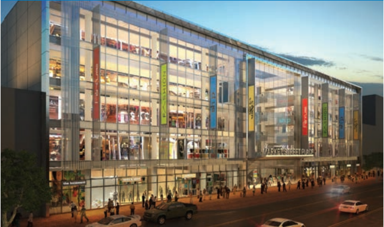
Market Street Place (image courtesy of CRP/Cypress Market Street, LLC)
