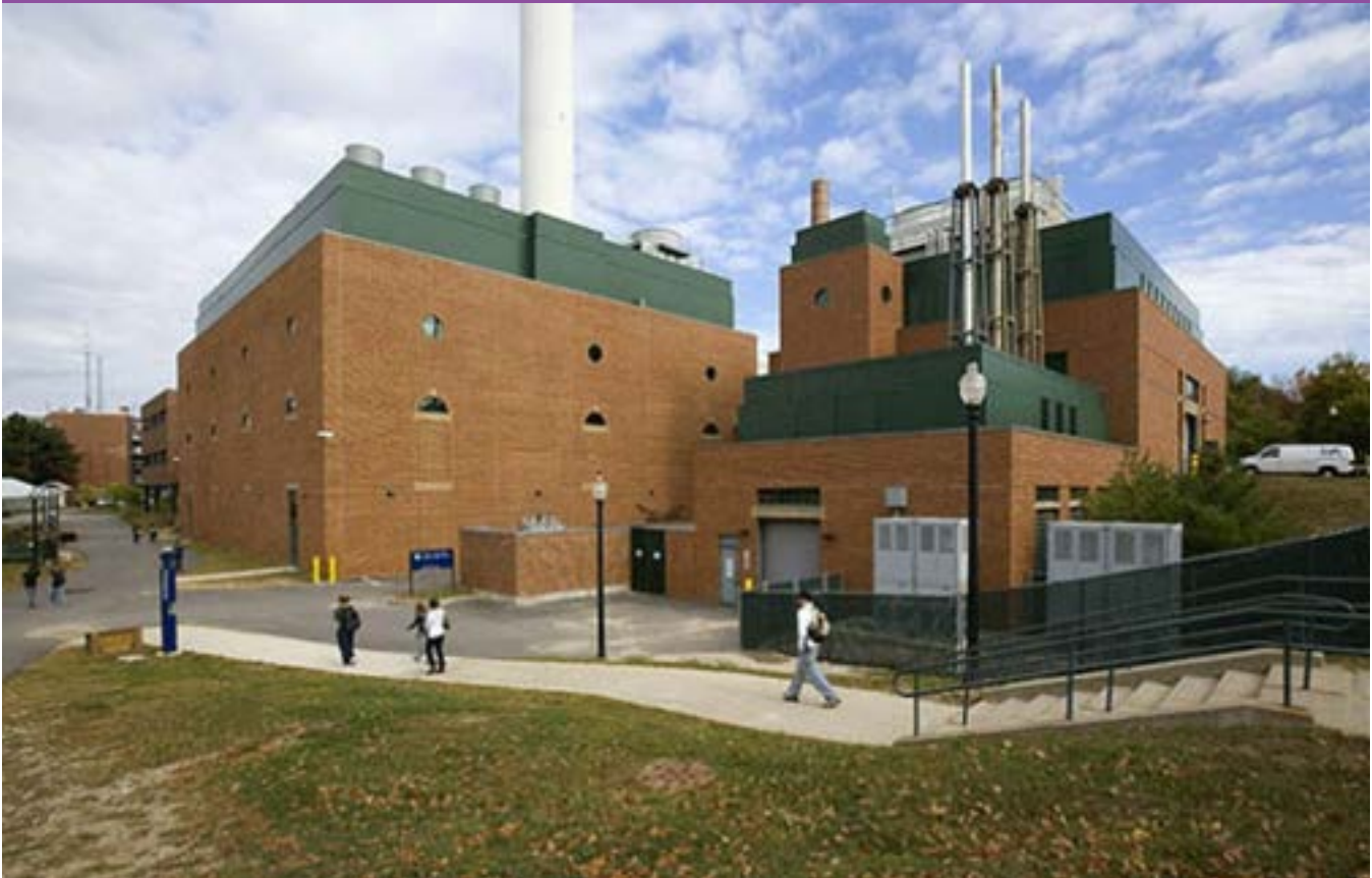
UConn Central Utilities Plant
