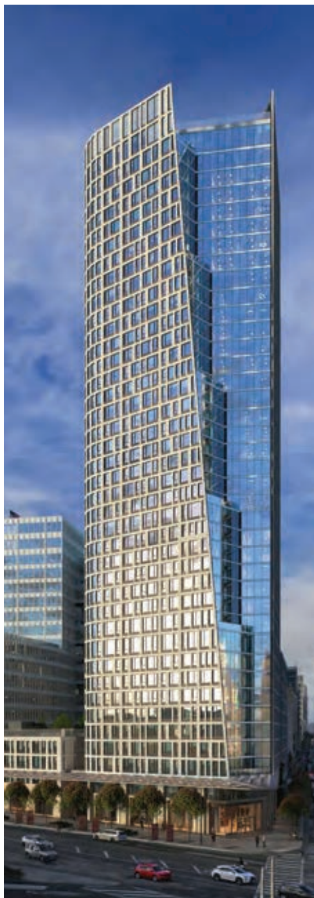
Fifteen Fifty, a high-rise residential tower in San Francisco, CA is reusing graywater and rainwater for toilet and urinal flushing and irrigation. (image courtesy of Epic Cleantec)
