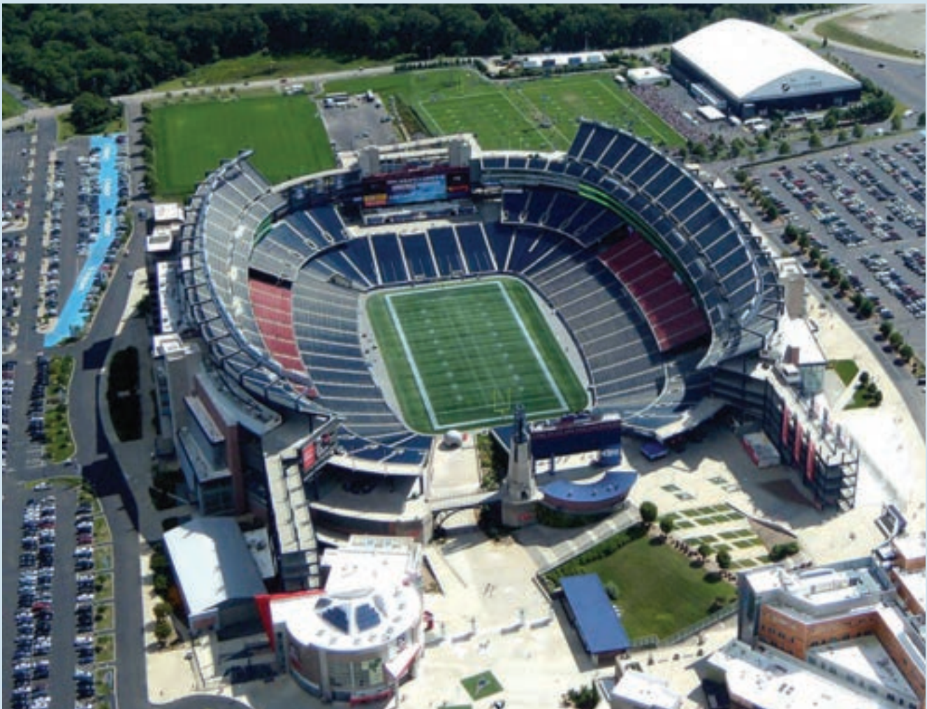
Gillette Stadium (image courtesy of Natural Systems Utilities)
