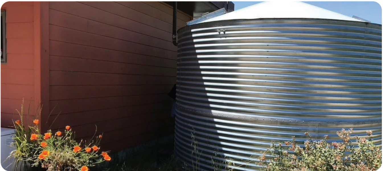
The EcoCenter at Heron's Head Park is showcasing sustainability with its own solar energy system, living roof, and onsite rainwater harvesting.
