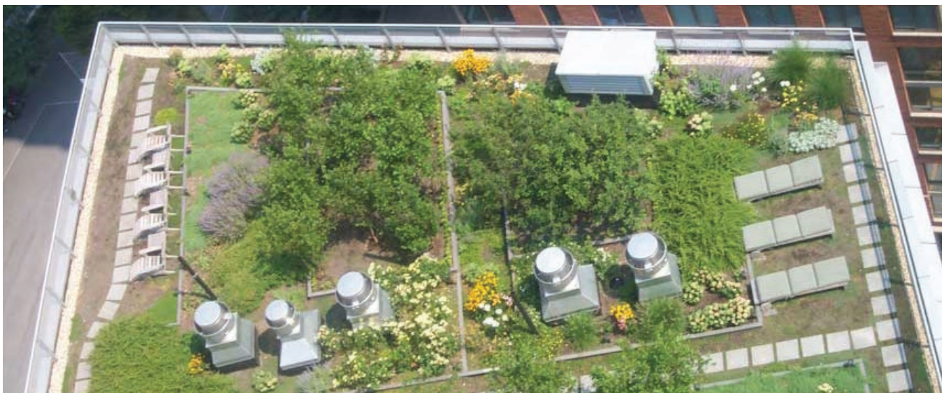
The green roof reduces runoff, insulates the building, and is irrigated by the onsite reuse system (image courtesy of NSU)
