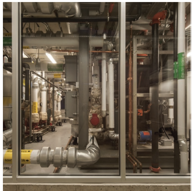
Onsite reuse system (image from Gray & Osborne Inc., Consulting Engineer’s Bullitt Center Water Treatment System Engineering Report)
