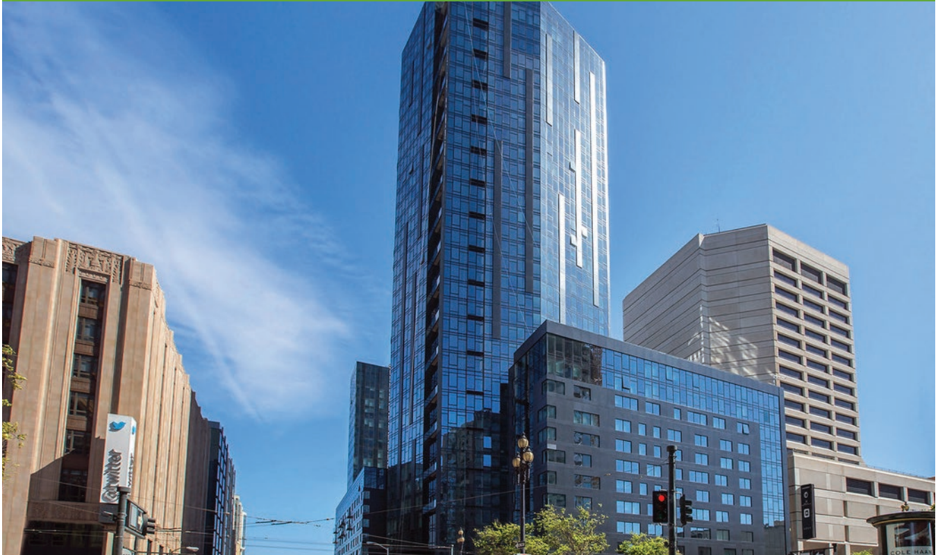
NEMA apartment complex (image courtesy of Epic Cleantec)
