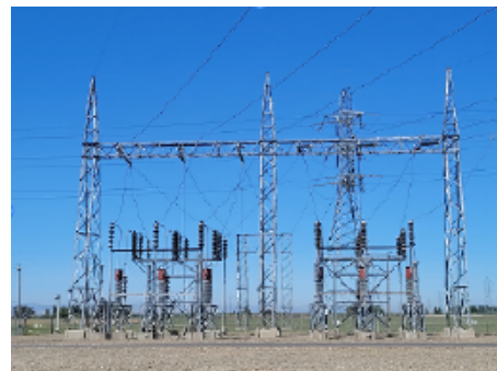
Warnerville Substation Rehabilitation - Phase 2 South Yard PG&E Tie-in
