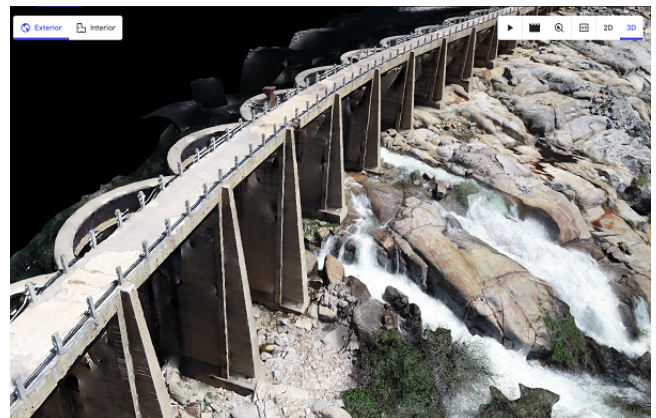
Lake Eleanor Dam - A Multiple Arch Reinforced Concrete Dam
