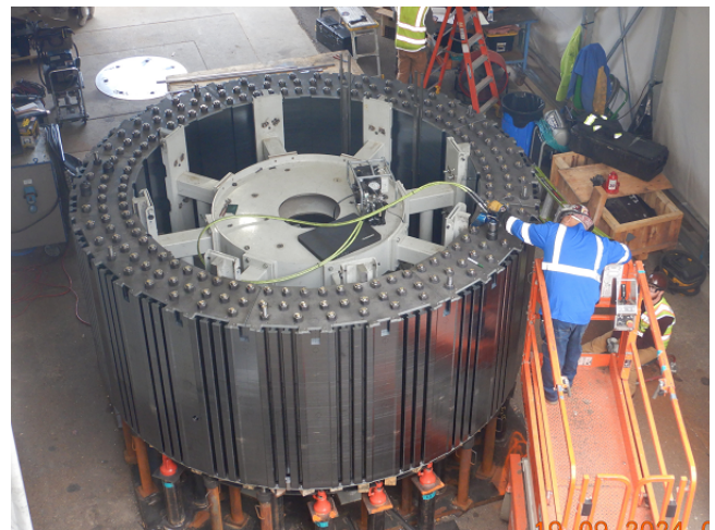
Checking Rotor Bolt Elongation after Torquing
