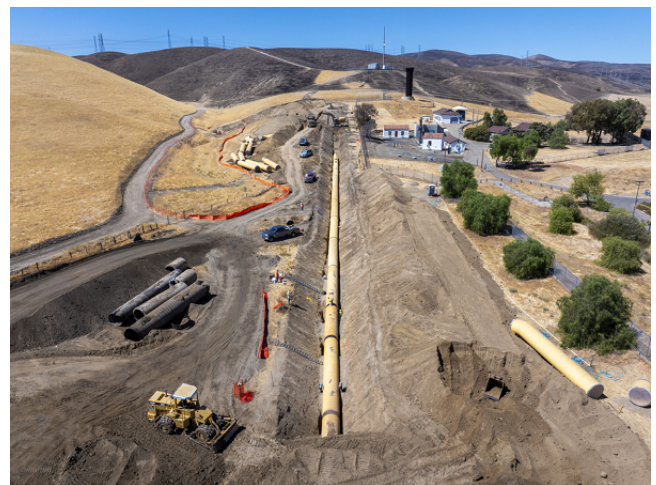
60-inch Pipes Being Laid at Tesla Surge Tower Site
