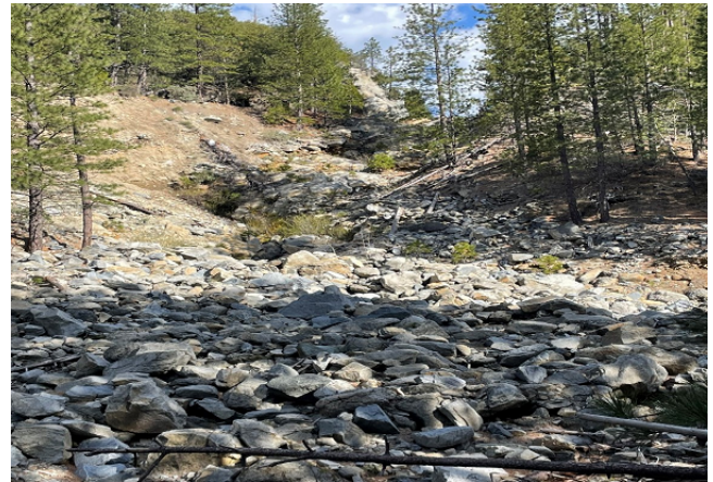
Erosional Channel in the Project Area, Facing North
