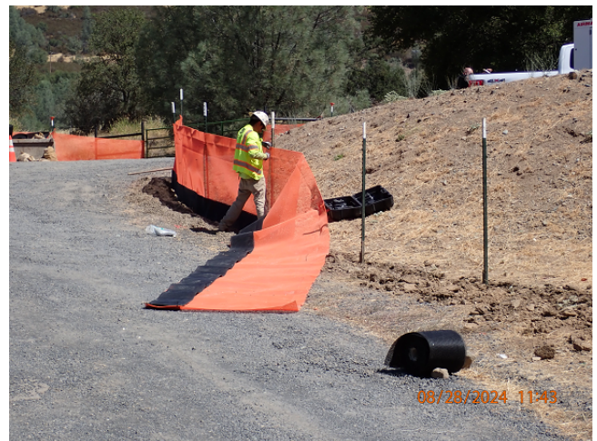
Contractor Mobilized to the Site (August 2024)
