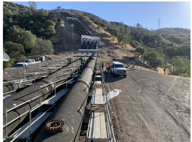
Scaffolding Setup to Conduct Phased Array Ultrasonic Testing
