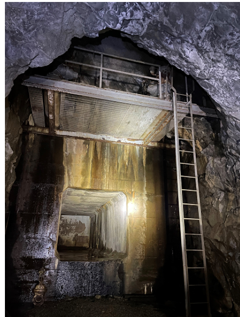
Canyon Tunnel - Hetchy Adit Bulkhead
