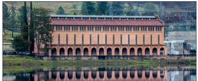
Existing Moccasin Old Powerhouse
