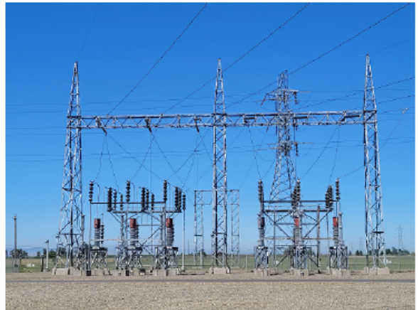
Warnerville Substation Ph 2 South Yard PG&E Tie-in Upgrade
