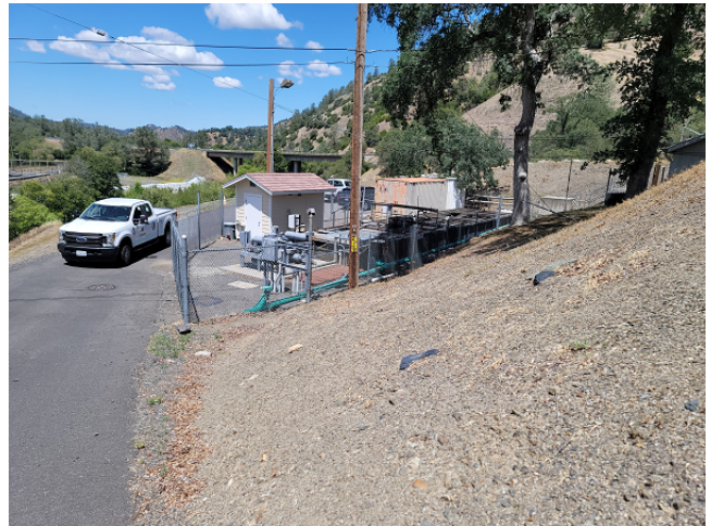
Existing Moccasin Wastewater Treatment Plant
