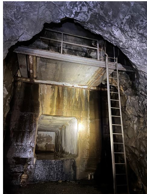
Canyon Tunnel - Hetchy Adit Bulkhead
