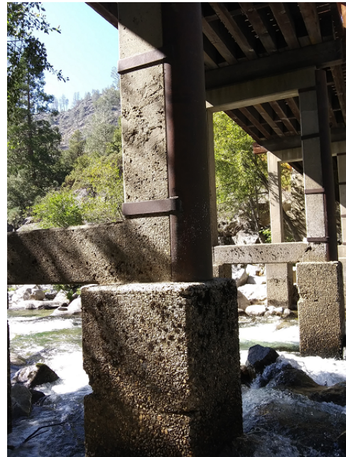
Concrete Footings and Piers of the O'Shaughnessy Adit Access Bridge
