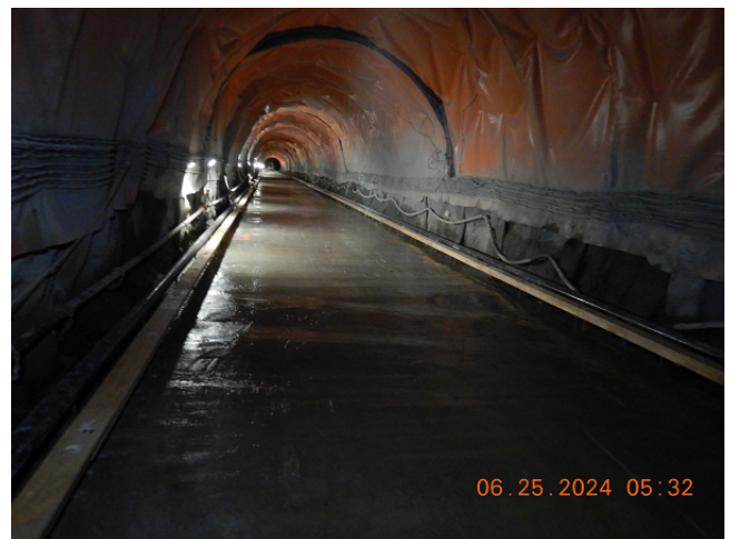
Priest Adit with Concrete Invert
