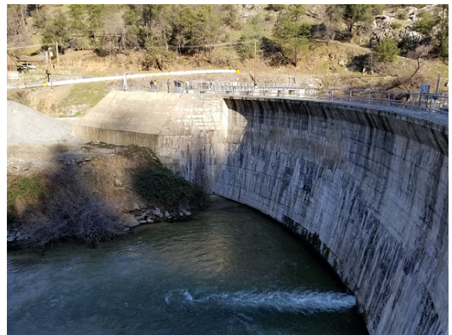
Early Intake Dam - Downstream side
