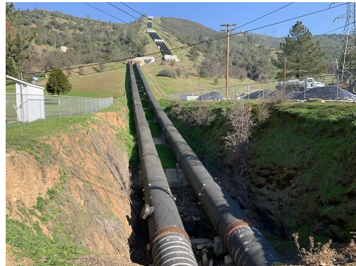
Moccasin Penstock along steep section
