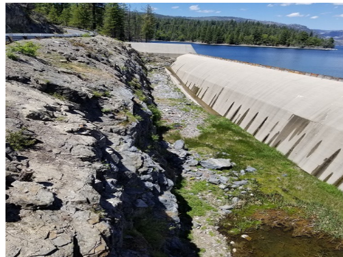
The Spillway Overflow Weir and Upstream Channel
