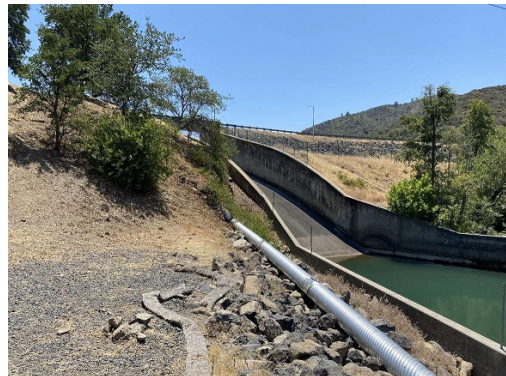
Existing Moccasin Dam Spillway
