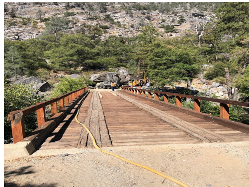
O’Shaughnessy Adit Bridge and Geotechnical Exploration
