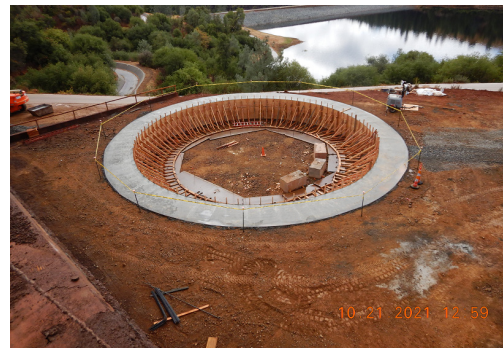
FCF Shaft Collar Construction
