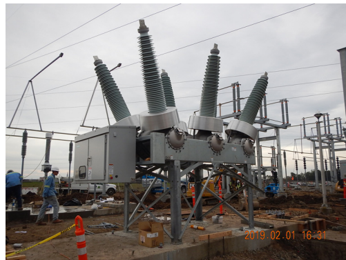
Typical 230KV SF6 Breaker to be Installed as Part of Phase 2
