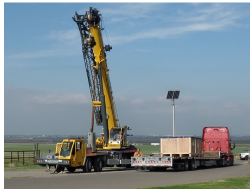
Delivery of 66-Inch Butterfly Valve to the Tesla Facility
