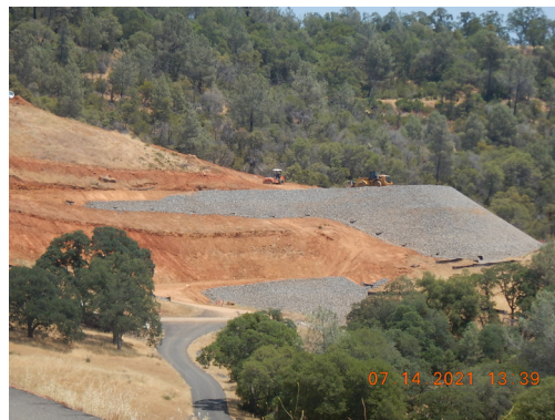
Priest Spoils Disposal Site Development underway
