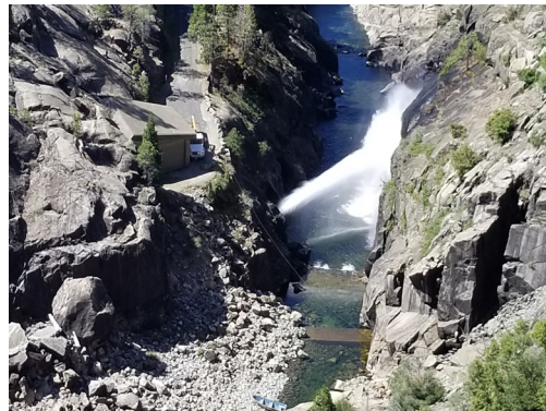
Discharge from the Instream Flow Release Valve
