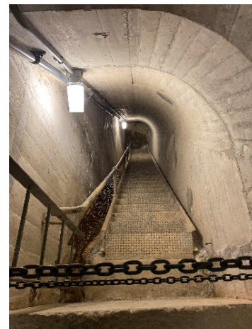
Inclined Stairway OSH Dam
