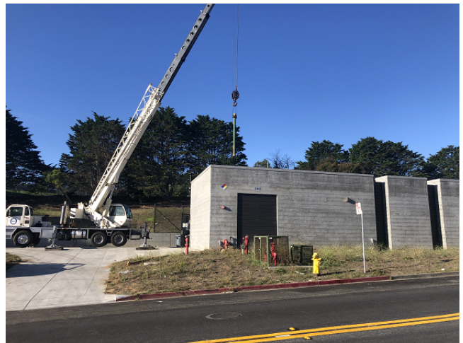
Column pipe removal for well rehabilitation at Colma BART Well Station
