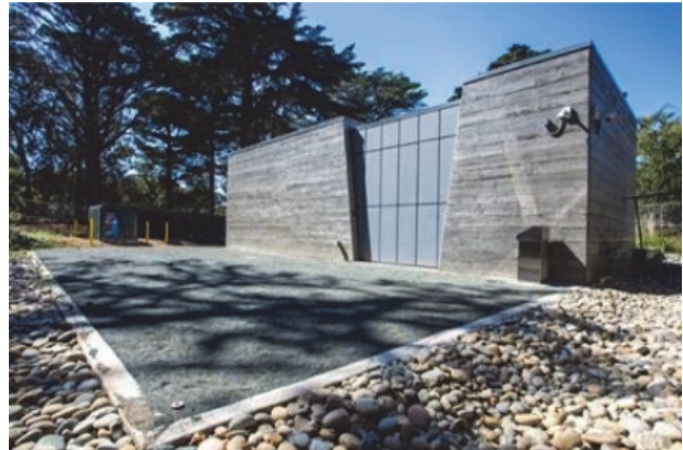
North Lake Well Station
