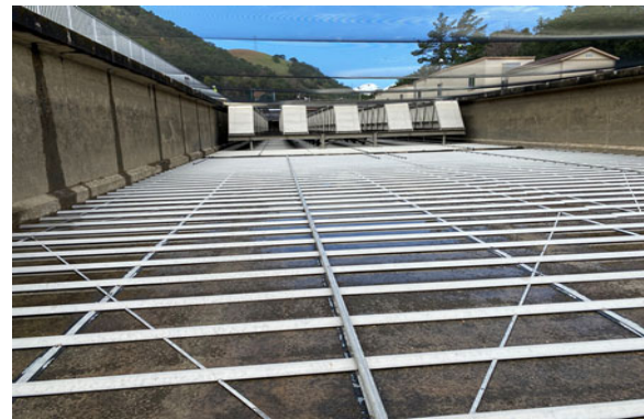
Inspection of Sedimentation Basin 1
