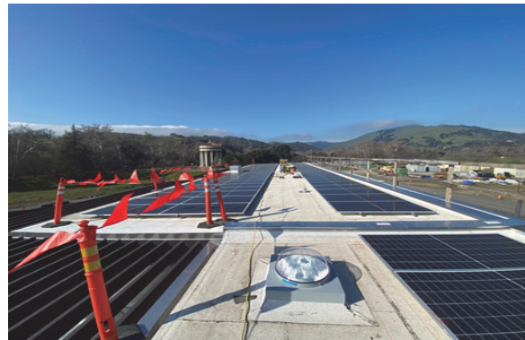
Installation of Solar Panels and Skylight on Roof
