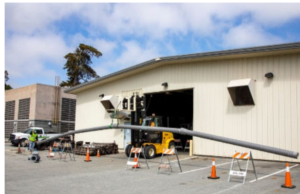
Earthquake Resistant Ductile Iron Pipe with flexible joints (demonstrated) used in the project
