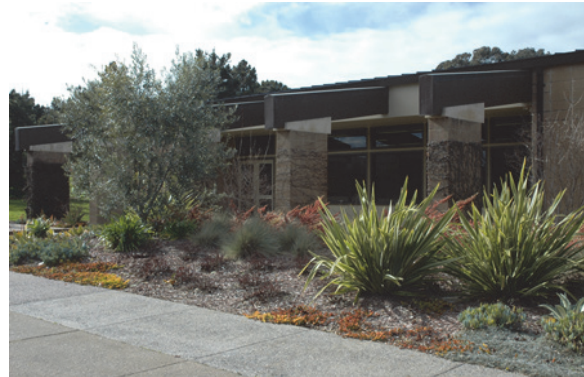
Existing Administration Building
