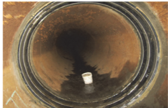
Typical Internal Pipeline Repair with WEKO Seals
