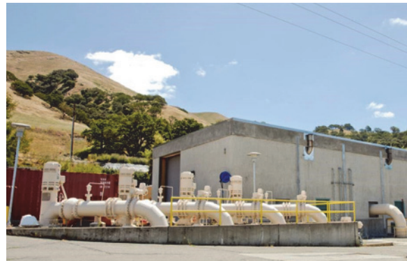
San Antonio Pump Station building looking southeast
