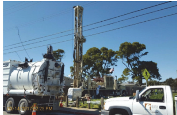
Deep Anode Installation – Corrosion Phase 1
