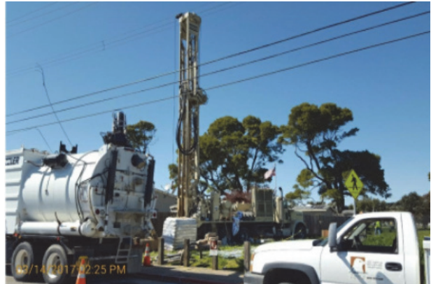
Deep Anode Installation – Corrosion Phase 1
