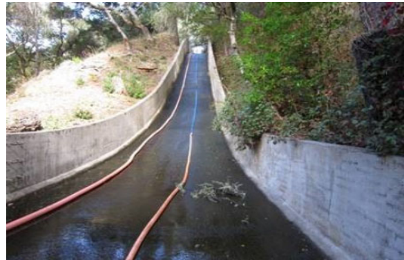
Spillway cleaning and mapping for condition assessment
