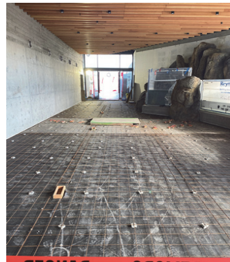
Exhibition Hall – Topping Slab Preparation
