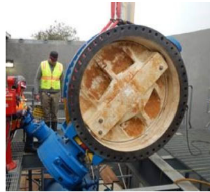
Typical butterfly valve to be installed for pipeline safe entry
