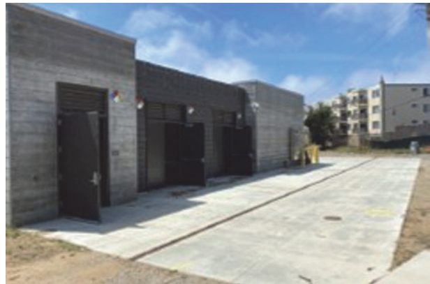
Well Station Building
