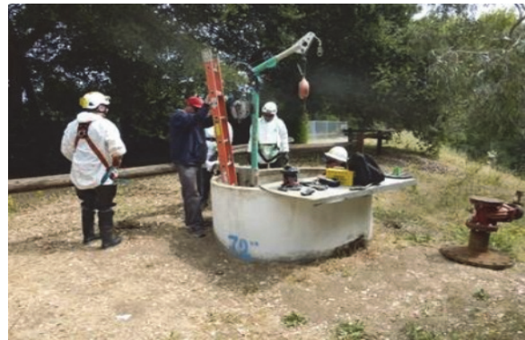
Typical Pipeline Entry for Inspections
