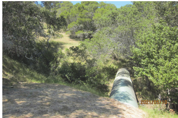
CSPL2 Gully Crossing
