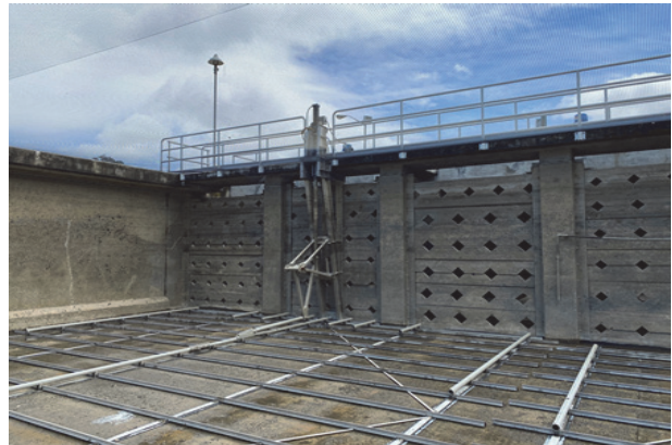
Inspection of Sedimentation Basin 1
