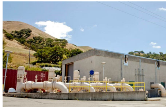
San Antonio Pump Station building looking southeast
