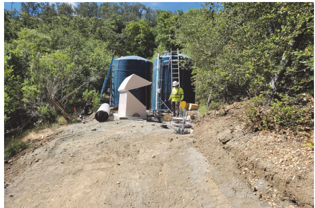
Installation of hypochlorite system at High Valley tanks
