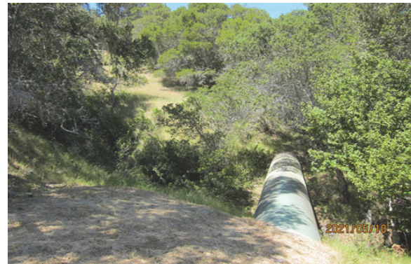
CSPL2 Gully Crossing with Limited Vehicle Access
