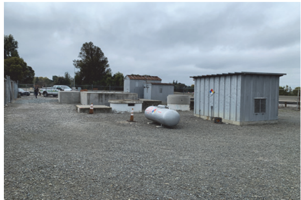
Valve Lot Where New Valve Will be Added for Safe Entry
