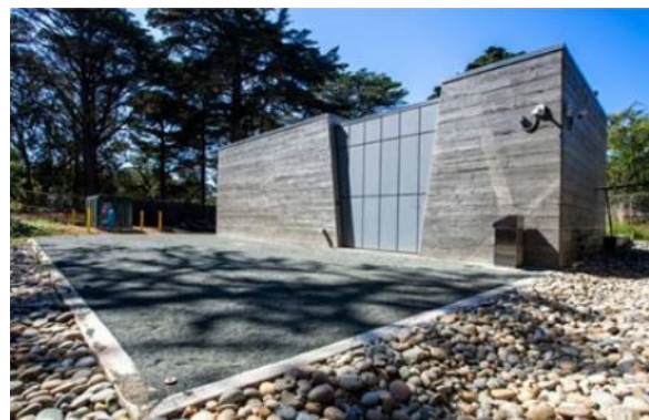
North Lake Well Station
