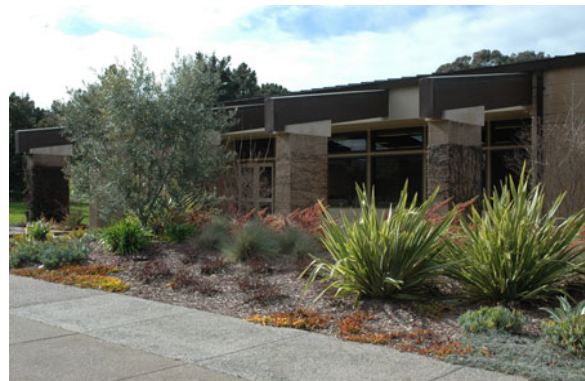
Existing Administration Building
