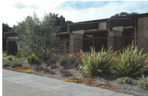
Existing Administration Building
