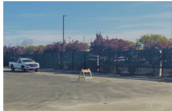
View of newly installed fence on north property line
