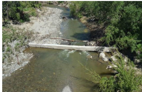
Exposed Town of Sunol Pipeline crossing Arroyo de la Laguna Creek
