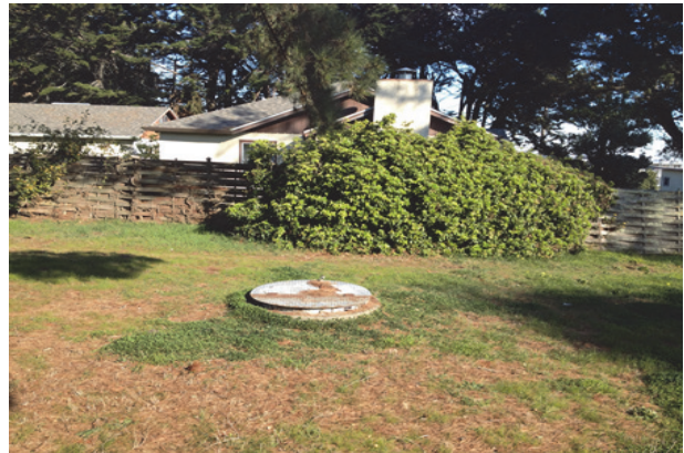
Typical Appurtenance to be Upgraded
