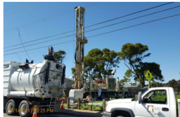
Deep Anode Installation – Corrosion Phase 1
