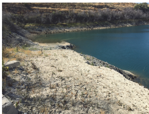
Current Condition of Pond F2 Access Road
