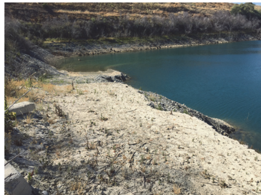
Current Condition of Pond F2 Access Road
