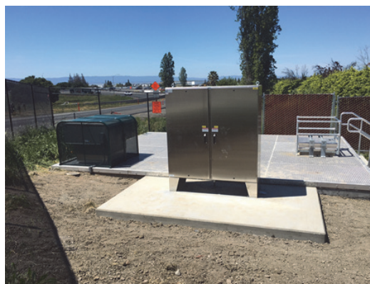
Ventilation and Sump Pump Project
