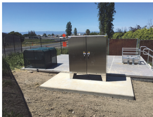
Ventilation and Sump Pump Project
