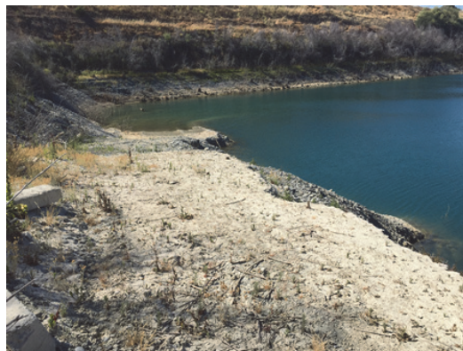
Current Condition of Pond F2 Access Road
