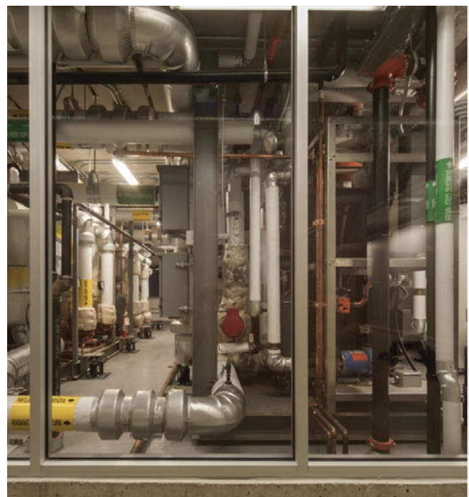
Onsite reuse system (image from Gray & Osborne Inc., Consulting Engineer's Bullitt Center Water Treatment System Engineering Report)
