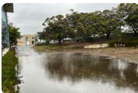
EXISTING SITE PHOTOS
