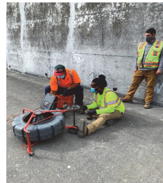
Sub-Drain Inspection at the Turner Dam Spillway
