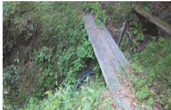
CSPL2 alignment along creek bank
