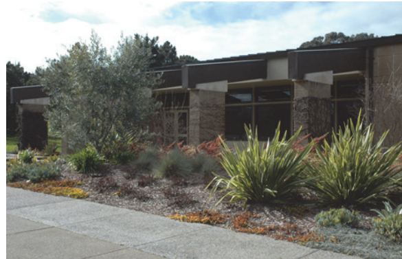
Existing Administration Building
