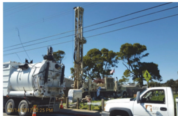
Deep Anode Installation – Corrosion Phase 1
