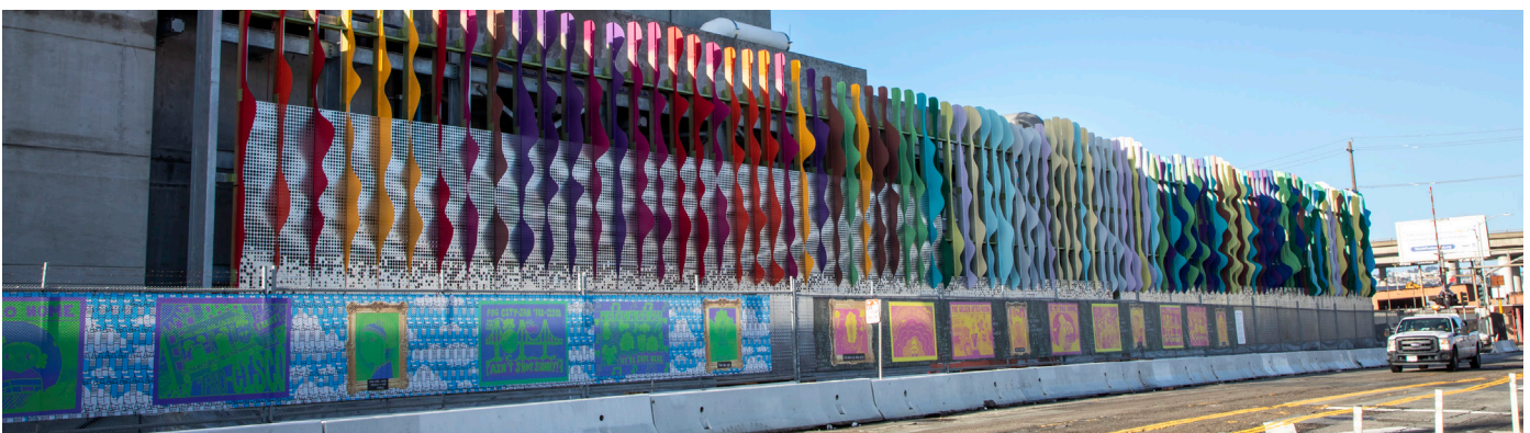
“Whorl Whirl: Our Circular Nature” by artist Norie Sato, is the 335-feet long and 35-feet high permanent art installation on the Southeast Treatment Plant wall on Evans Avenue.
