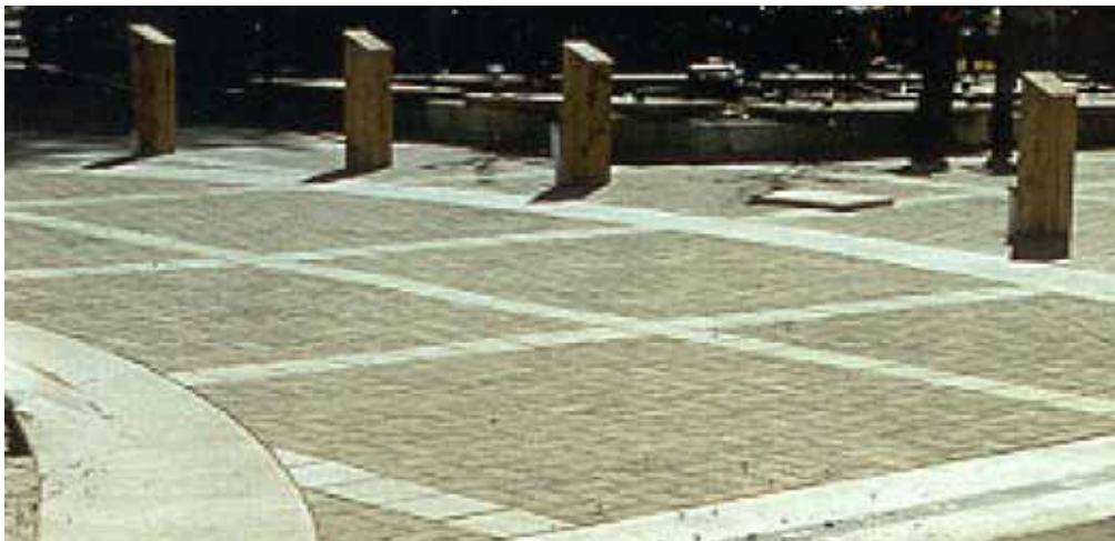
Permeable pavement can be integrated into a variety of hardscapes such as roads and sidewalks, plazas, terraces and patios.
