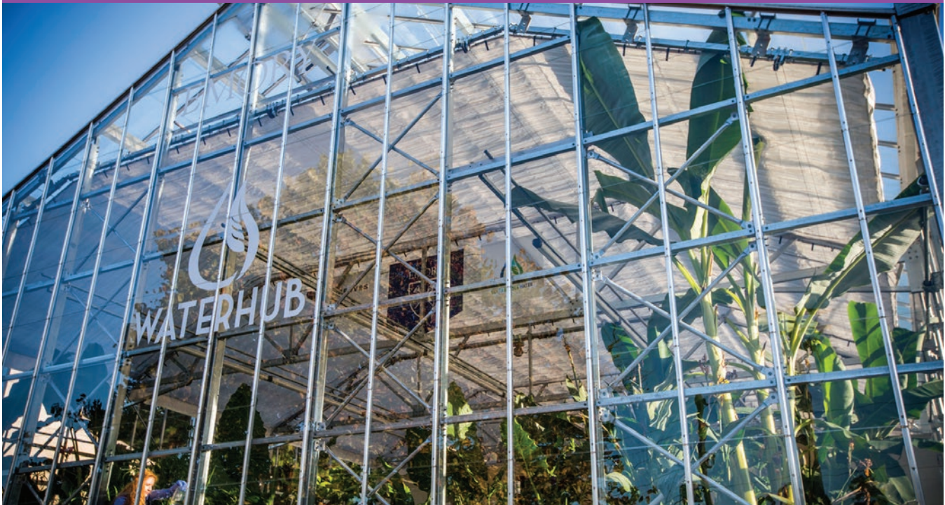
Exterior of the WaterHub greenhouse at Emory University (image courtesy of Sustainable Water)
