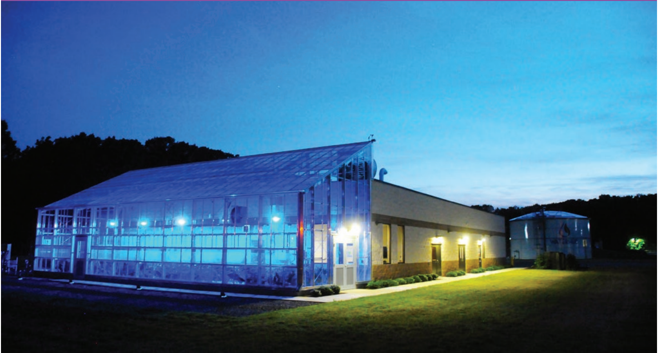
The WaterHub's greenhouse, administrative building, and reclaimed water storage tank (image courtesy of Sustainable Water)
