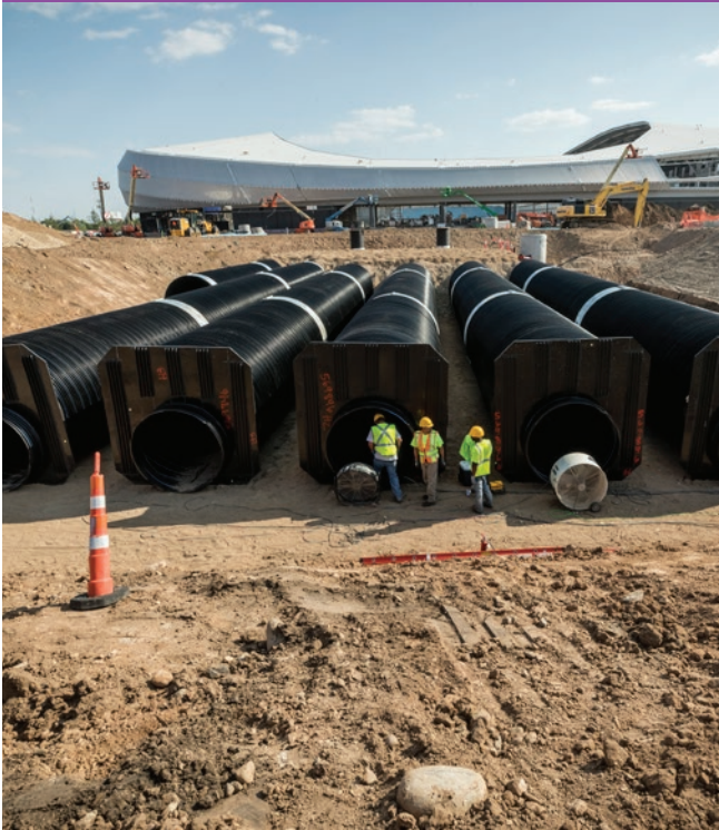
Installation of underground rainwater storage tank outside of stadium (Image courtesy of the City of St. Paul)
