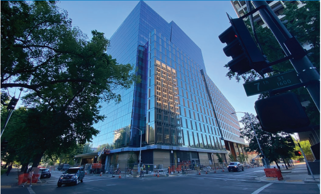
DGS Natural Resources Building under final stage of construction (image courtesy of HTEC)
