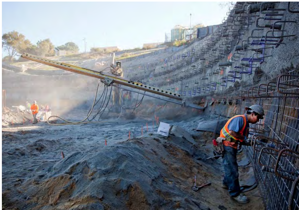
FIGURE 19 - HTWTP PROJECT SITE
