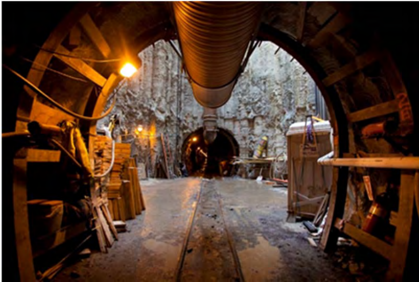
FIGURE 27 NEW IRVINGTON TUNNEL PROJECT SITE
