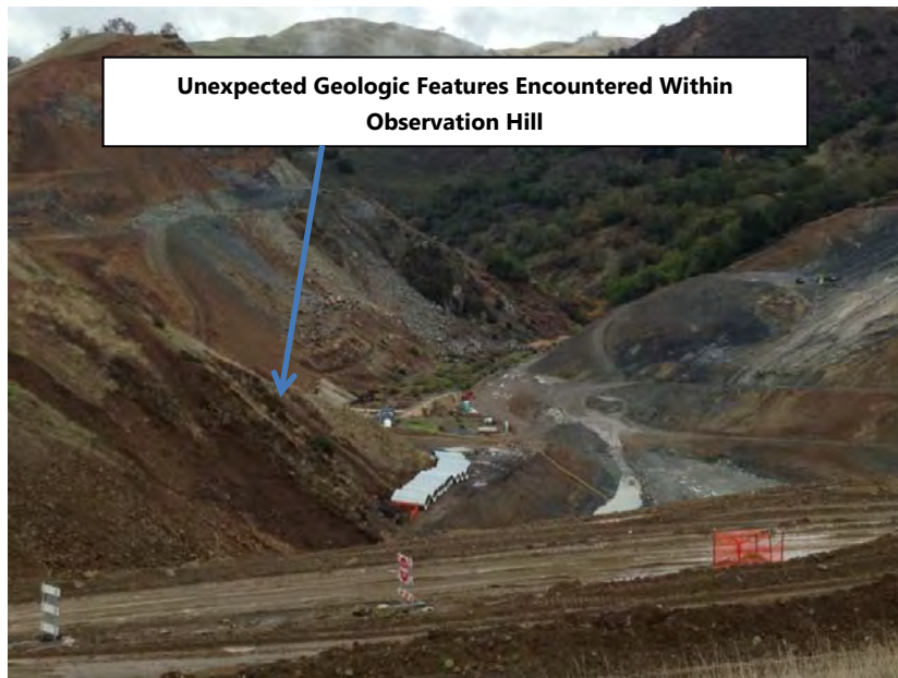
FIGURE 5 - FIELD PHOTOGRAPH OF ENCOUNTERED CONDITION
