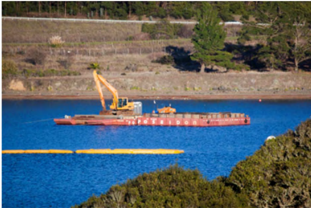
FIGURE 12 - CSSA PROJECT SITE - MARINE CONSTRUCTION
