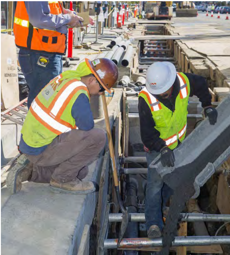
BCTD Project construction in Mission Bay
