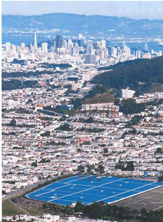
Solar Panels at Sunset Reservoir
