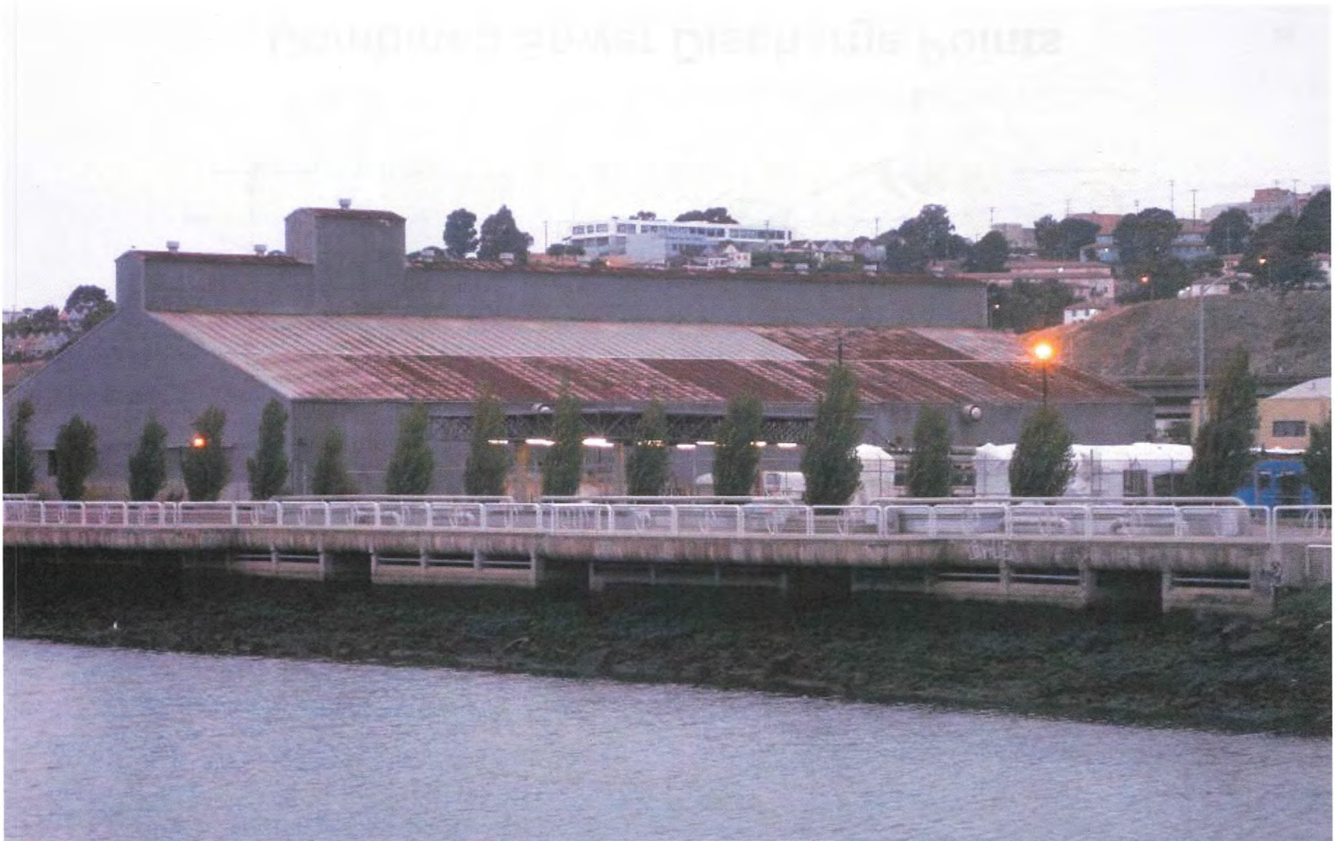
Islais Creek North Discharge Structure
