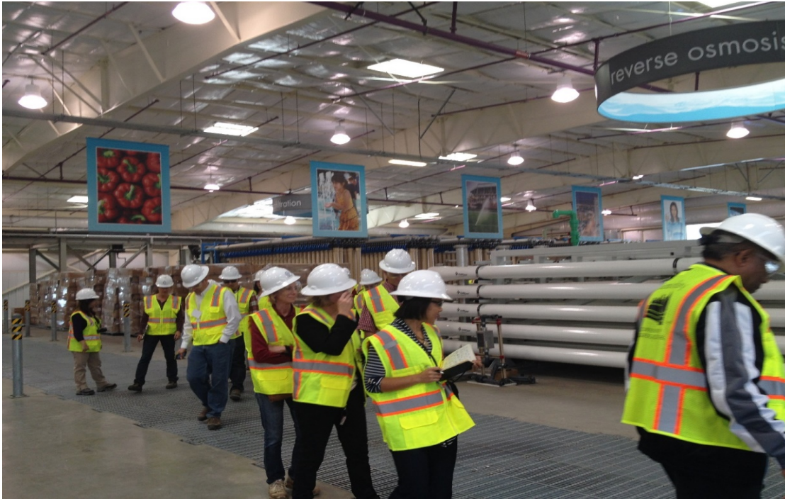
Figure 3.3 Silicon Valley Advanced Water Purification Center in San Jose, California
