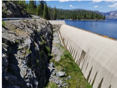
Cherry Valley Dam Spillway
