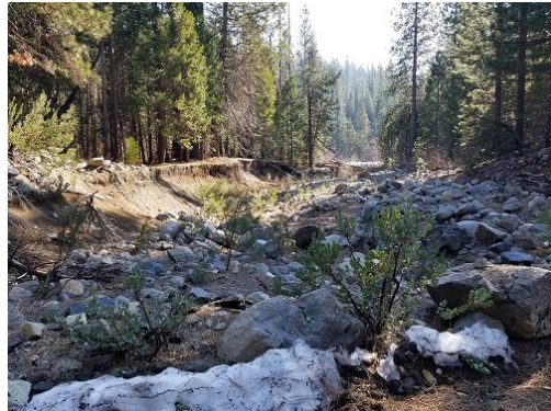
Cherry Valley Dam Spillway Downstream Channel (looking downstream)
