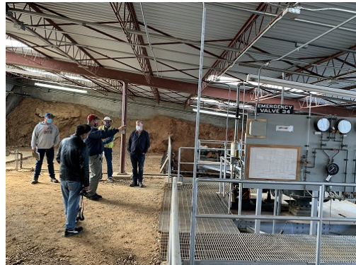
Site visit inside West Portal Valve House
