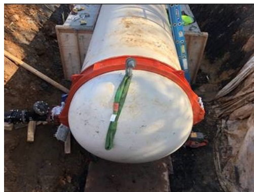
Construction Photo of a Victaulic Cap and Coupling SJPL 1 @ Oakdale
