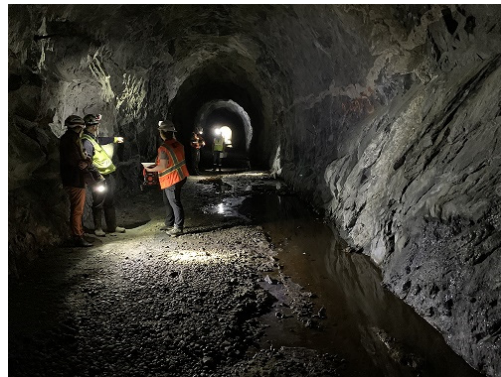
Site visit to evaluate the existing plug at Hetch Hetchy Adit within the Canyon Tunnel.
