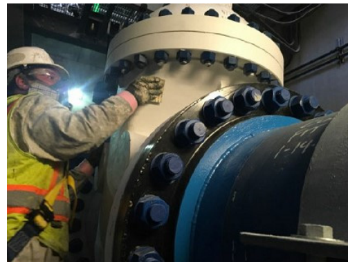
Worker performing coating repair for the 24-inch butterfly valve
