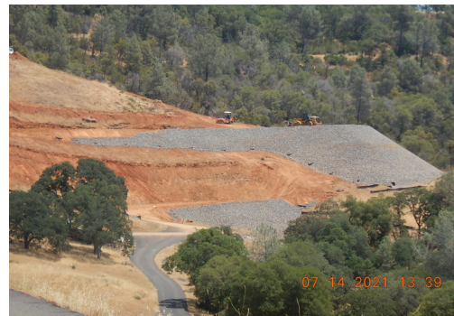
Priest Spoils Disposal Site Development underway
