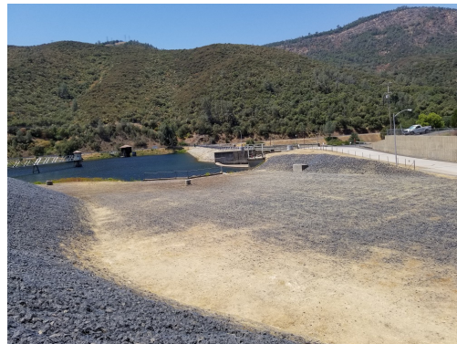
Moccasin Dam Upstream Entrance to Existing Auxiliary Spillway (looking upstream)
