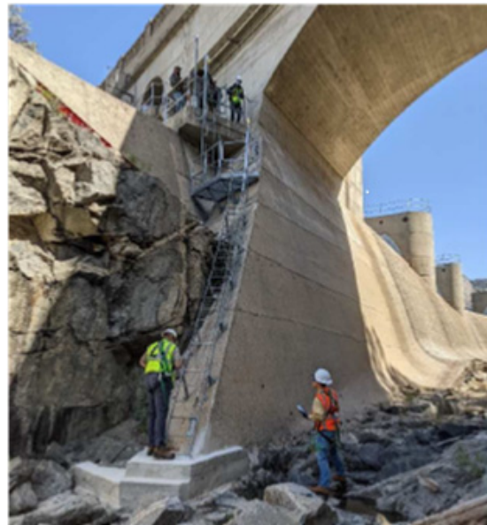
Exterior Ladder and Fall Protection to Spillway Invert
