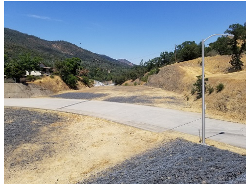
Moccasin Dam Existing Auxiliary Spillway
