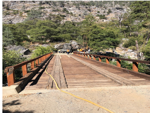
O’Shaughnessy Adit Bridge and Geotechnical Exploration
