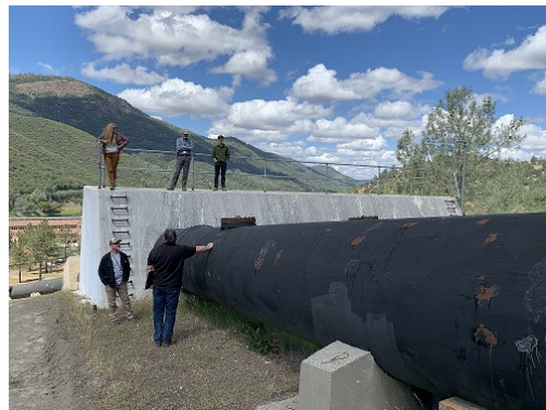
Site visit to evaluate the Moccasin penstock manway openings
