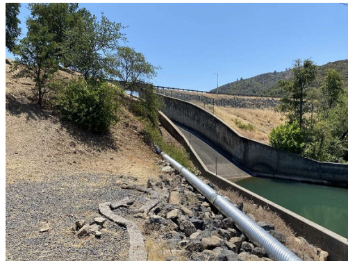
Existing Moccasin Dam Spillway
