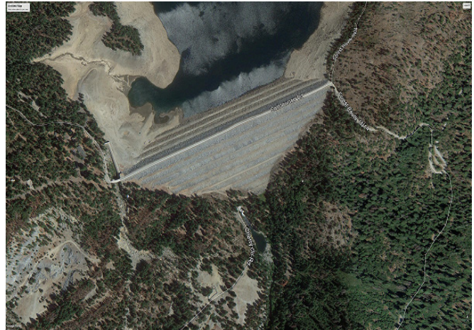
Cherry Valley Dam and Spillway
