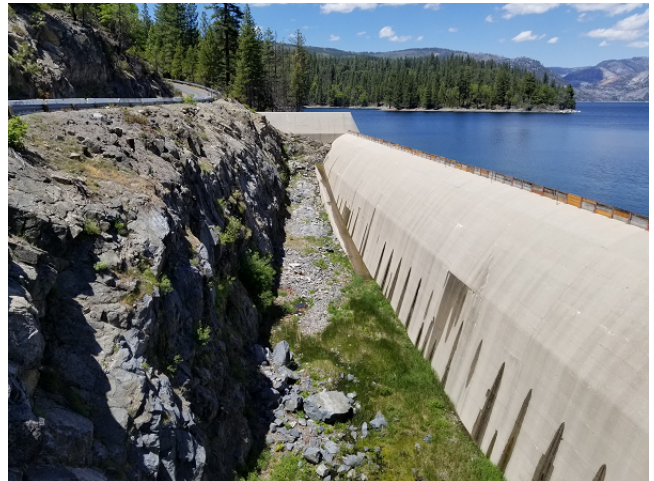
Cherry Valley Dam Spillway
