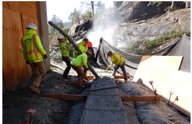
Concrete Footing Construction Outside of Diversion Tunnel Access Building
