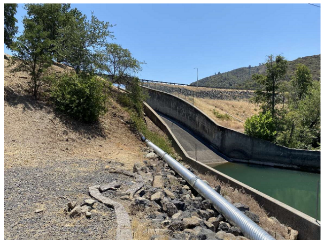
Moccasin Dam and Service Spillway
