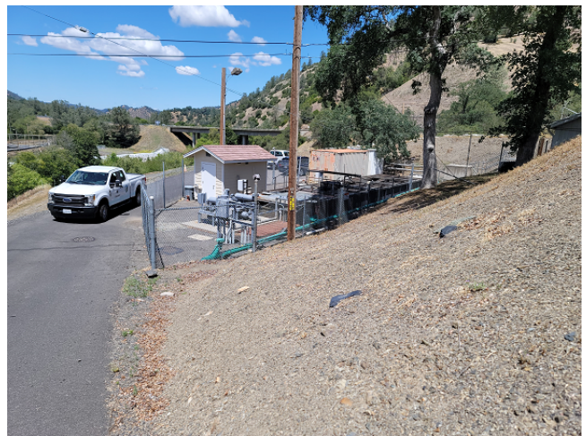
Existing Moccasin Wastewater Treatment Plant
