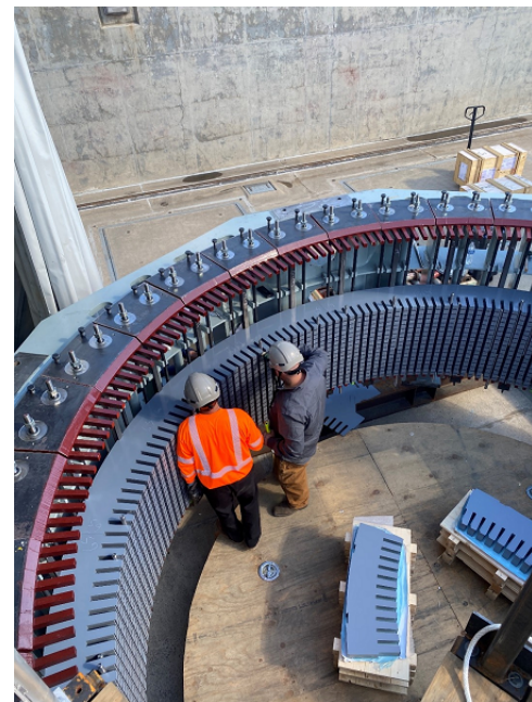
DB-121R2 Stator Frame being manufactured in Sorel-Tracy, Quebec
