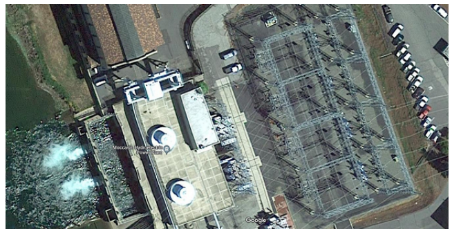
Existing Moccasin Switchyard
