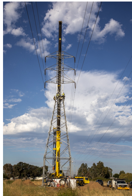
Tower 557S Raise - HH-1007 Transmission Line 7/8 Upgrades
