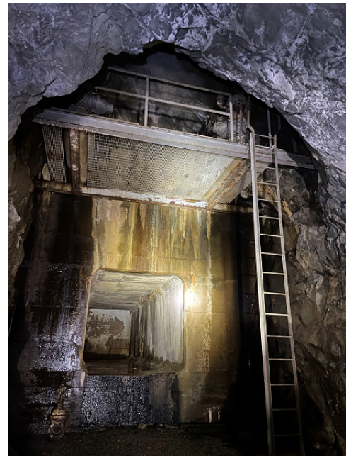
Canyon Tunnel - Hetchy Adit Bulkhead
