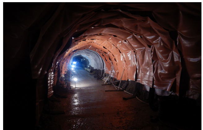
Inside the New Priest Adit showing Waterproofing Membrane
